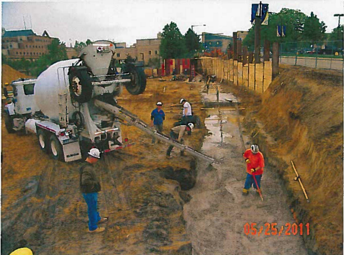
Wolf Ledges Engineering Building (Project# UAK100002) – Foundation pour
